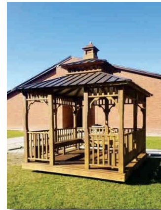
Double Roof With Cupola
